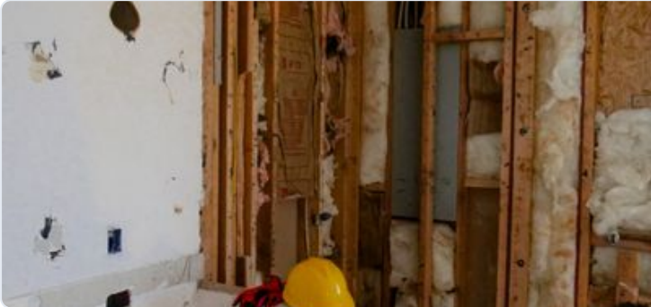
Ready for structural opening-up
