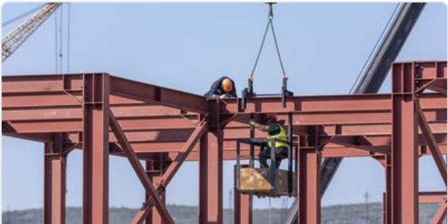
Progress photo — 17 Jul 2026
